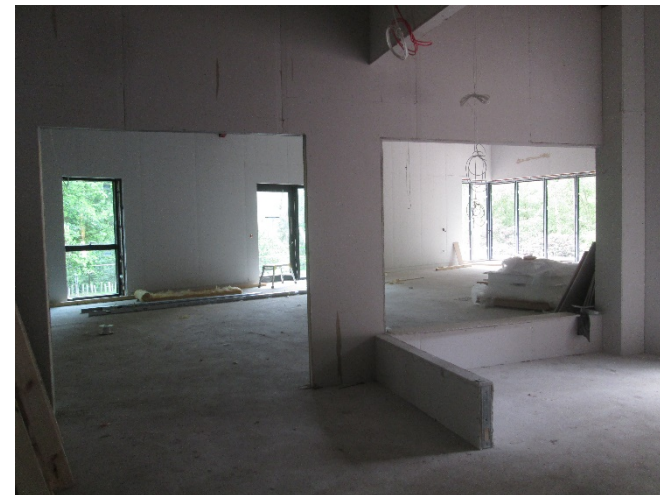
From entrance hall through to the activity room
